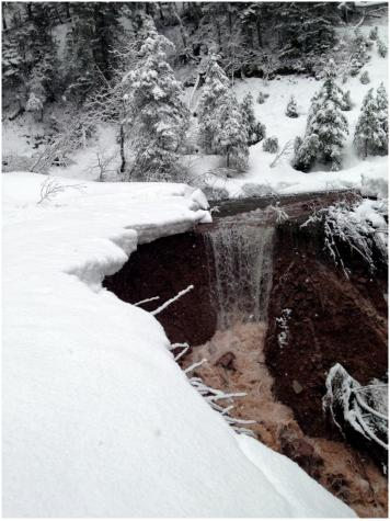
Figure 8: Substantial rain on snow caused damage on motorized access roads like this one on Pinnacle Road near Paola and Tunnel Creeks in the Middle Fork corridor of the Flathead Range.
